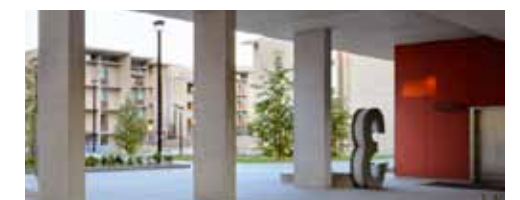
EXPRESSED CONCRETE STRUCTURE
