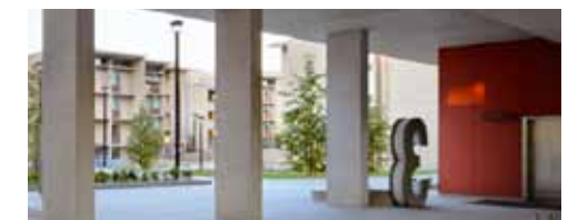
EXPRESSED CONCRETE STRUCTURE
