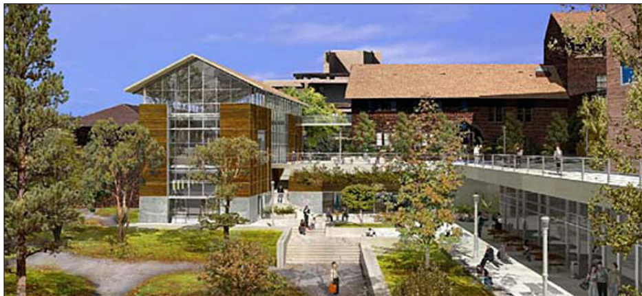
Blum Center and Naval Architecture Renovation
