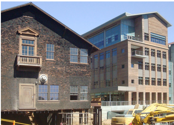
Naval Architecture (under renovation) and Sutardja Dai Hall
