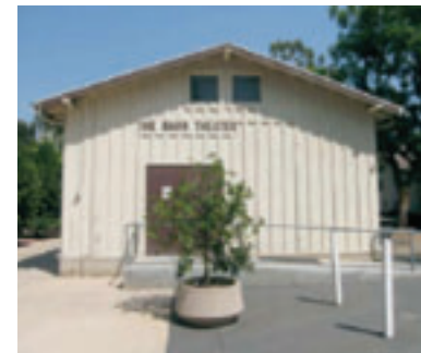
Barn Theater – West Façade
