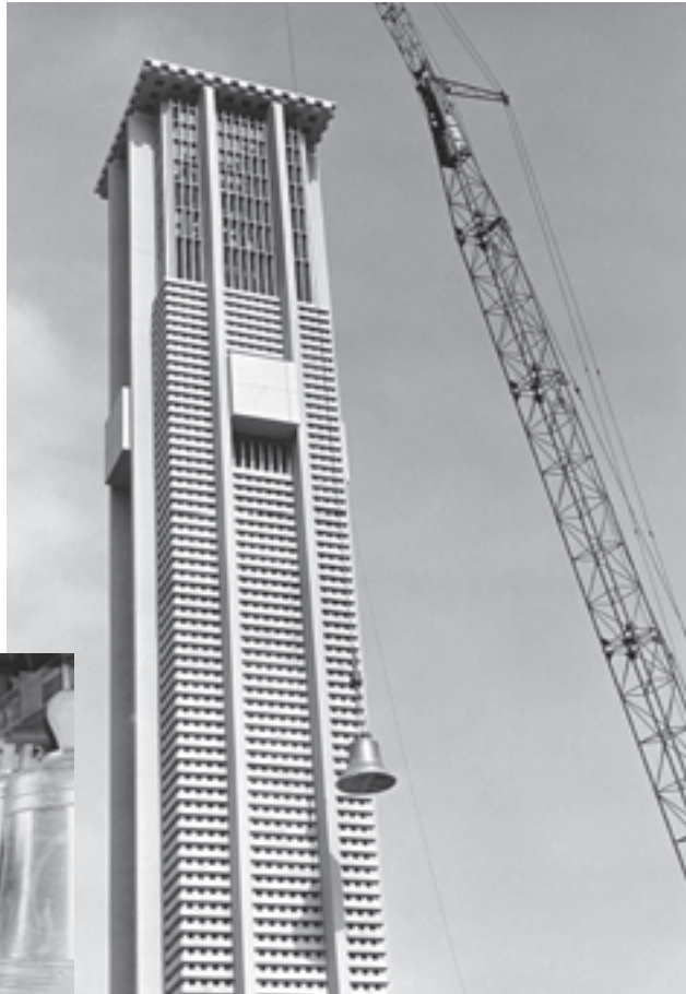
Construction of the Carillon Tower
