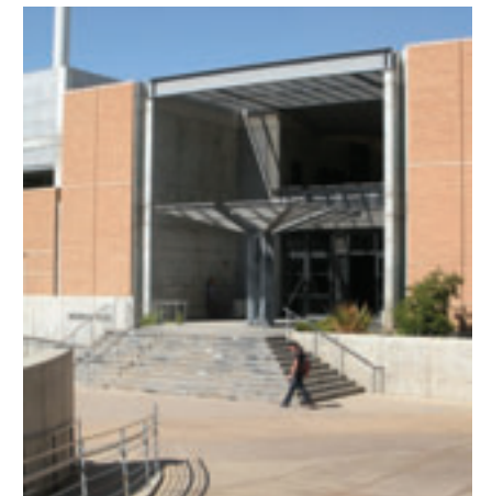
A Grand stairway and architectural recess announces an entry to Bourns Hall
