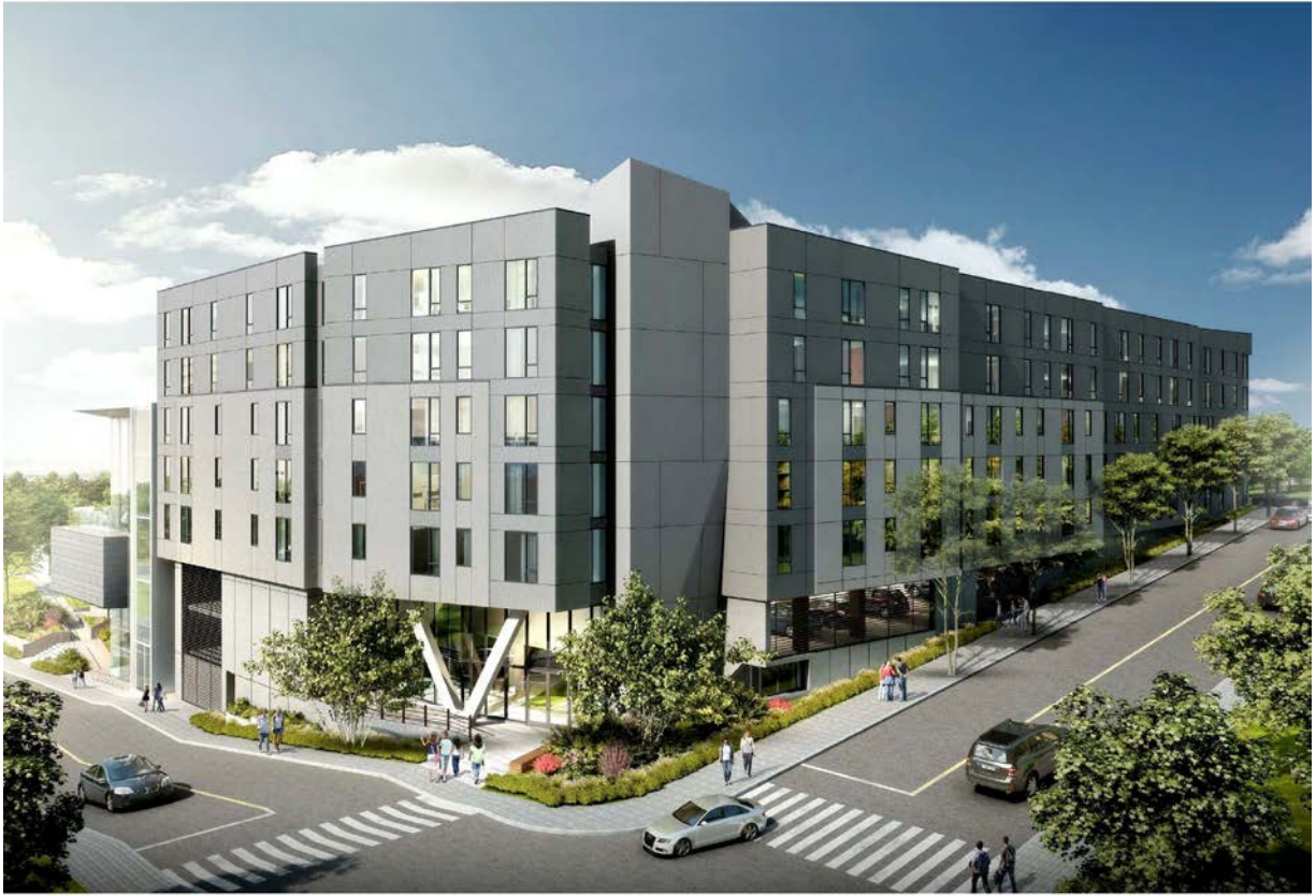
Residential Building, looking northwest from La Loma and Hearst Avenues
