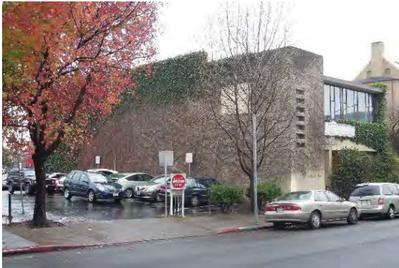
View looking southwest.
