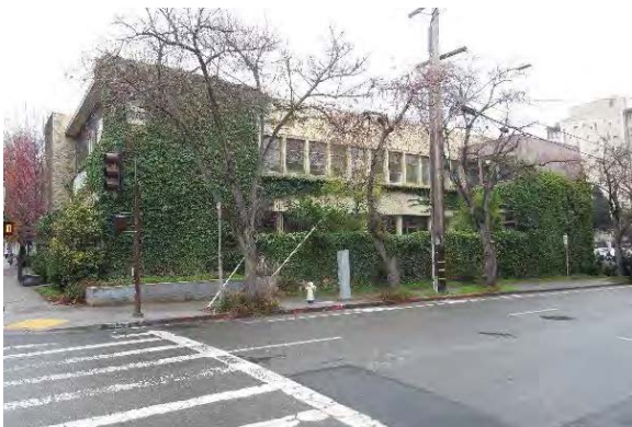
View looking east/southeast.
