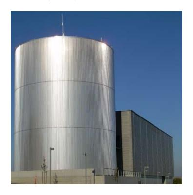
The campus' Central Plant is the first utility plant to ever receive a LEED Gold rating. It has also won local, state and national design awards. The Central Plant's two-million gallon thermal energy storage tank contains water that is chilled overnight for campus cooling purposes during the day. This saves energy and money for the campus.
