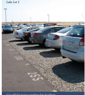
Geocellular porous parking lots facilitate stormwater capture and groundwater recharge.
