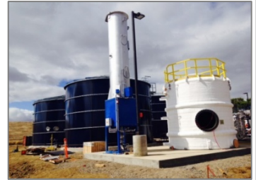
Completion of biodigester construction is scheduled for December 2013.
