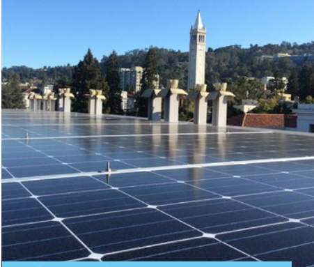
New solar installation on the roof of the MLK Student Union. Credit: Kira Stoll
