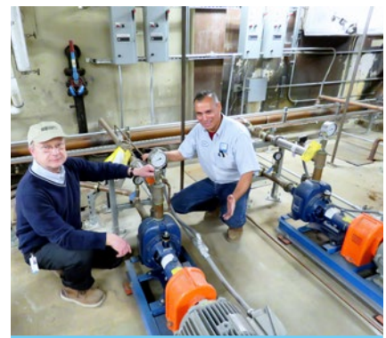
UCLA Facilities' employees Emilio Rodriguez and Giuseppe Scitutto work on the water efficiency project estimated to save 28 million gallons annually. Credit: Nurit Katz
